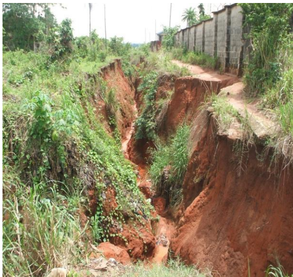
PLATE 1: Works layout road threatened by gully (source: authors field work 2016) Gully Erosion Development Process
